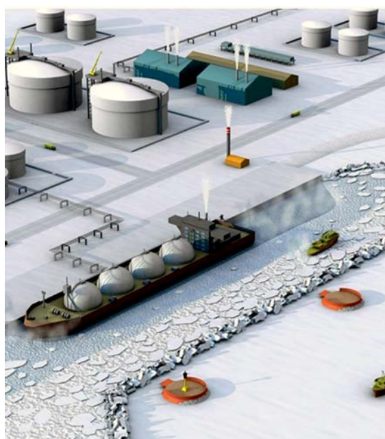
Arctic harbour design may include layout, planning of ship and icebreaker operations, brash ice control system and ice barrier design.
