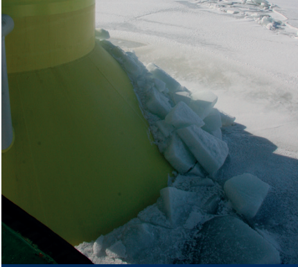
Results from model tests were used in the design and construction of the foundations at Tahkoluoto wind farm, the world’s first offshore wind farm built in a freezing sea. Photo: Suomen Hyötytuuli Oy
