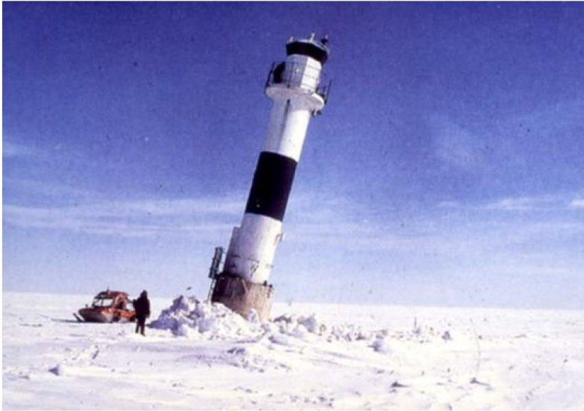
Lighthouse Bjørnklack after overloading event on 4th April 1985 (Engelbrektsen et al., 1987)
